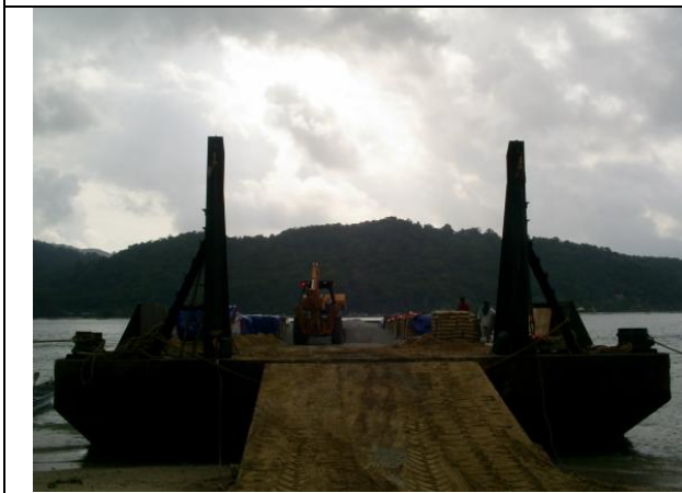
Materials being unload from barge at Pulau Perhentian
