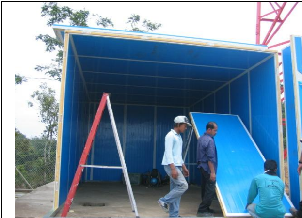
14' x 24' Cabin installation is in progress
