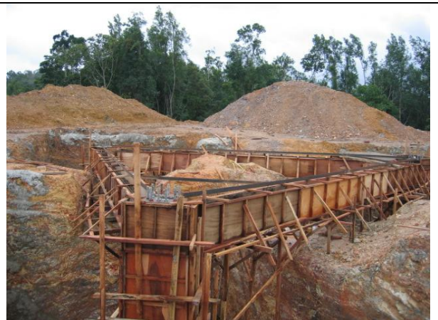
Tower foundation works are in progress at site.
