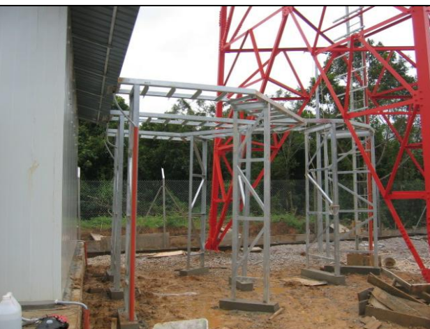
Cable gantry work is in progress.
