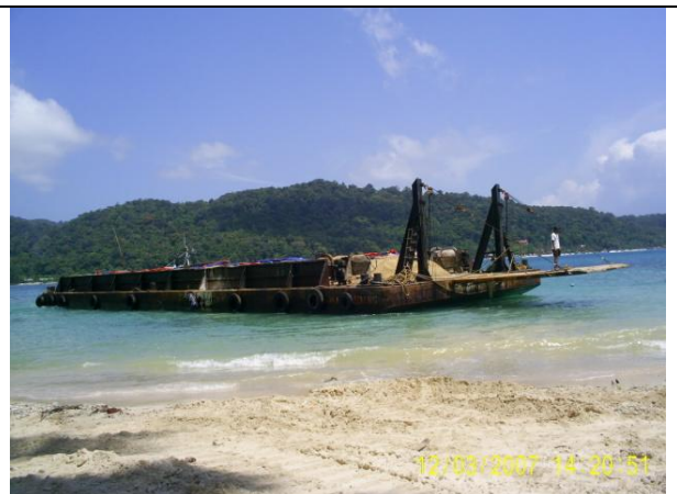
Transferring construction materials via 300 tones barge at Pulau Perhentian.
