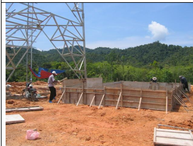
Workers preparing the formworks for the cabin plinth.
